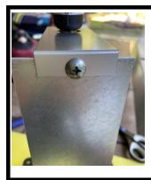
Set screw should be in place to secure the DBI bracket to the support bracket.
